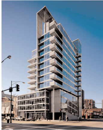
The Contemporaine condo high-rise at 516 N. Wells St. consists of a four-story parking garage topped by an 11-story residential tower.
