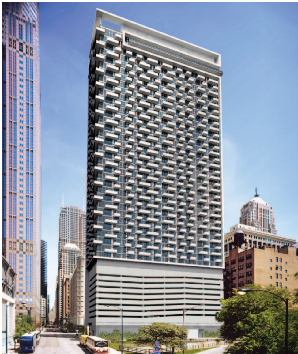
235 Van Buren, designed by award-winning architect Ralph Johnson
